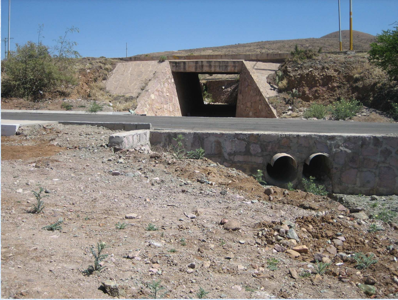
Figure 6. Photo of existing culverts.
